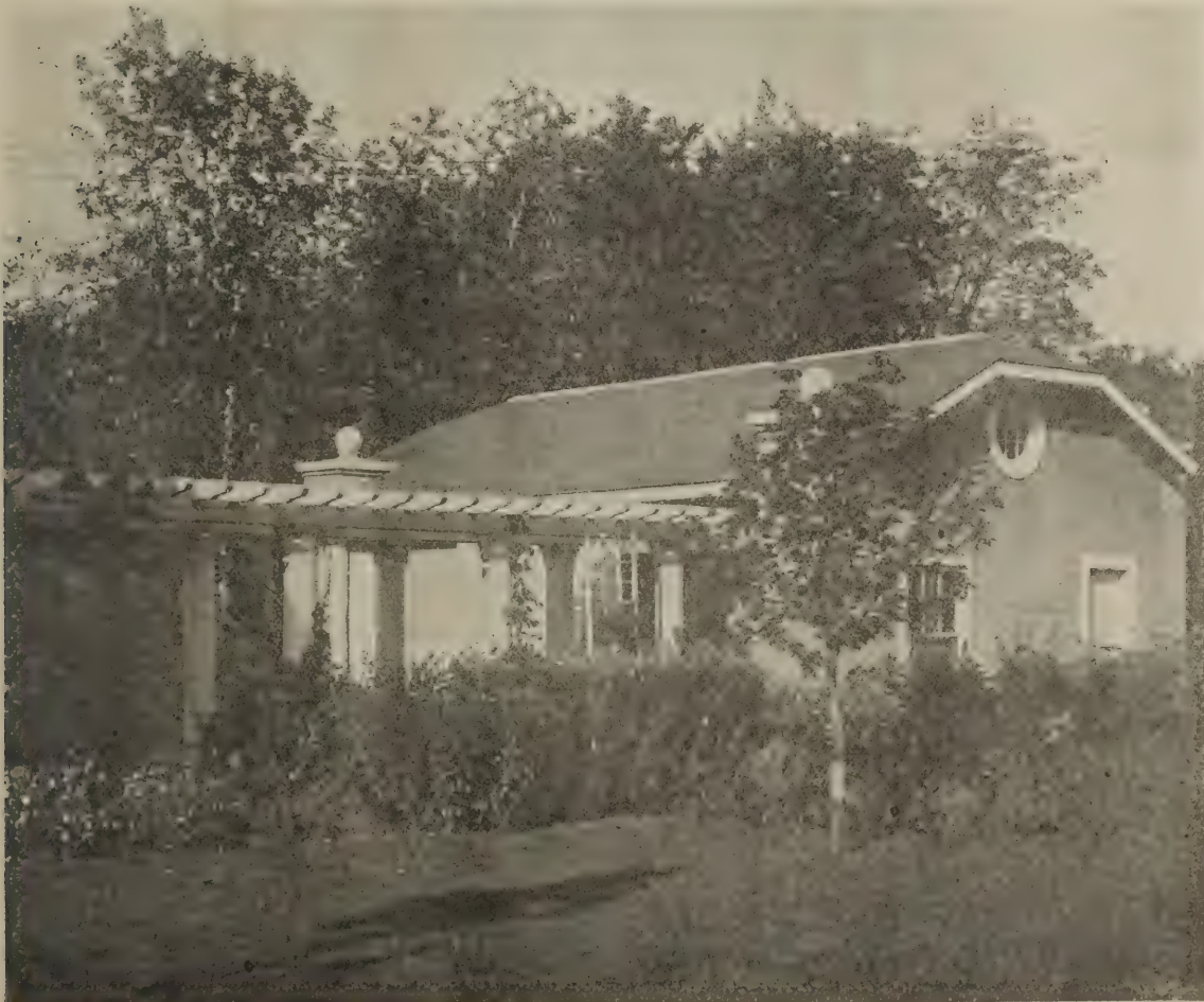
Garage with connecting pergola, at Oak Park, Ill.
